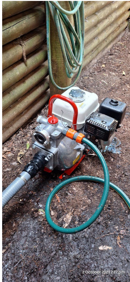
Portable Pump Under House + Storz & Hose to Sprinkler Outlets
